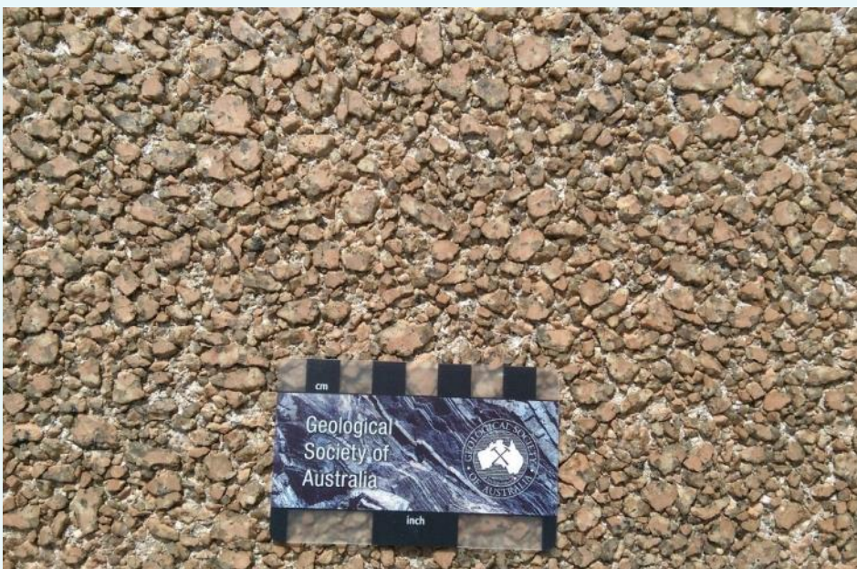
Detail of the huge polished aggregate slabs used in the walls of the Sydney Opera House, comprising abundant fragments of pink Tarana Granite. Photo courtesy Mike Smith.
