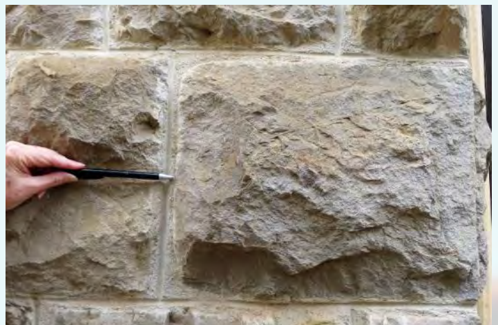
Black Mountain Sandstone blocks used to build Gungahlin Homestead. Image courtesy Mike Smith.
