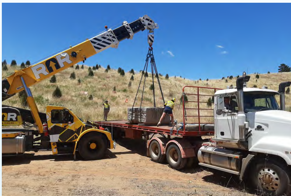
Placement of the large block from Eugowra in the NRG's temporary storage site in the Steering Committee's approved storage site in Canberra. Image courtesy Mike Smith.
