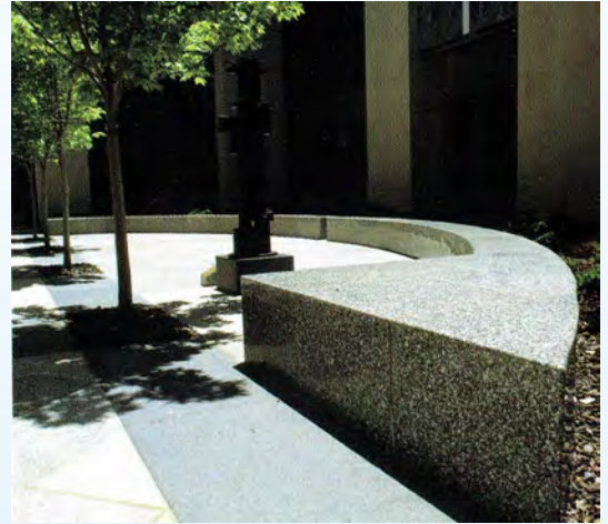
A low wall of Carmina Grey granite wraps around a courtyard on the Senate side of Parliament House. Image from Mayer 2009.
