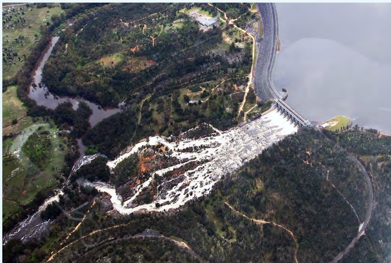
Wyangala Dam overflowing, 16 October 2022. Image courtesy Brad Pillans.
