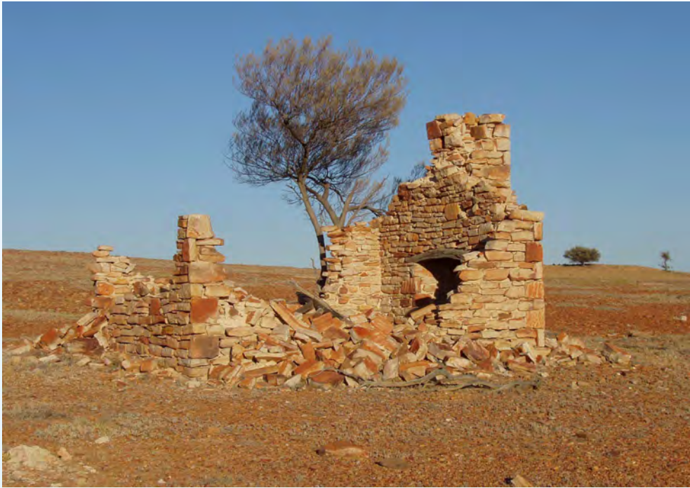
Figure 4. An abandoned stone cottage, built of silcrete, Stuart Creek, South Australia. Image courtesy B. Pillans.
