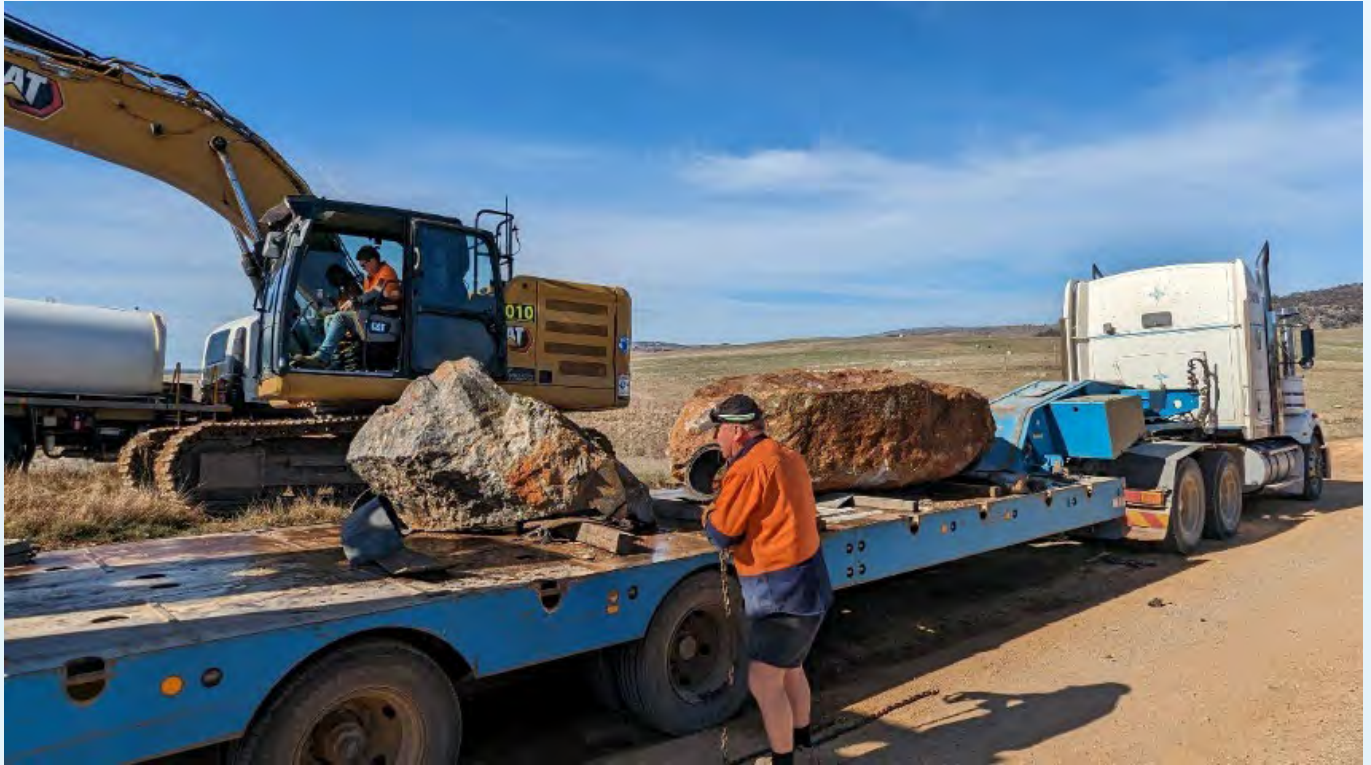
Men from the Snowy River – Monaro uploading two silcrete blocks at the Bobeyan Road cutting. Image courtesy Peter Fogarty.
